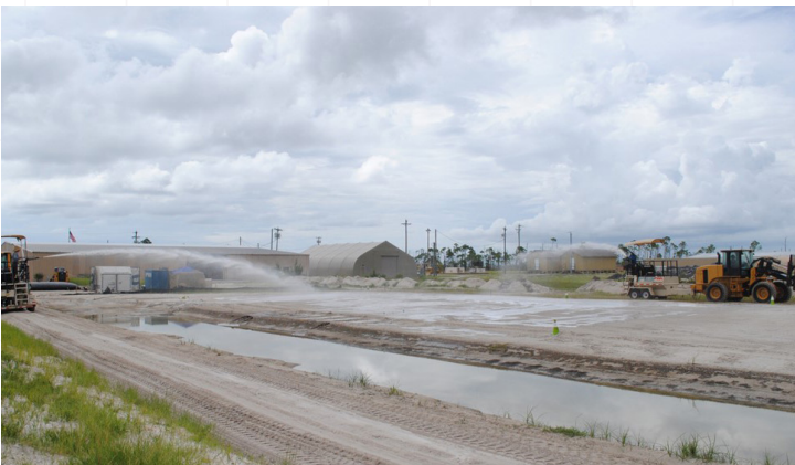
Biocement being sprayed on sandy soil at Tyndall, AFB. Photo Credit: Grace Bland
